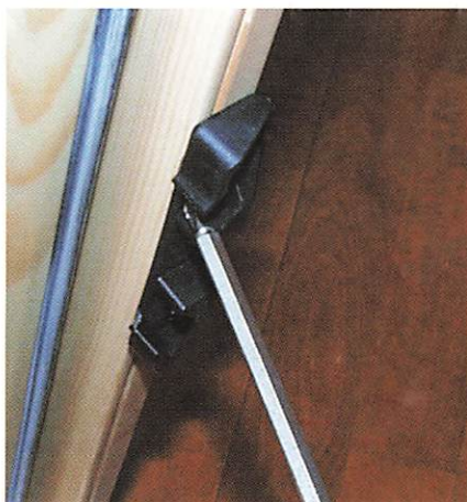
5 GGL ) Remove the GGL striking plate
