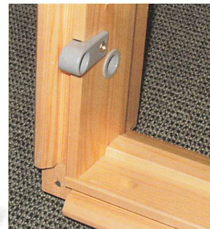
7 GGL ) Mount the barrel bolt bushing
